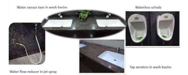
Photograph 7: Sensor based Taps at MIAL
